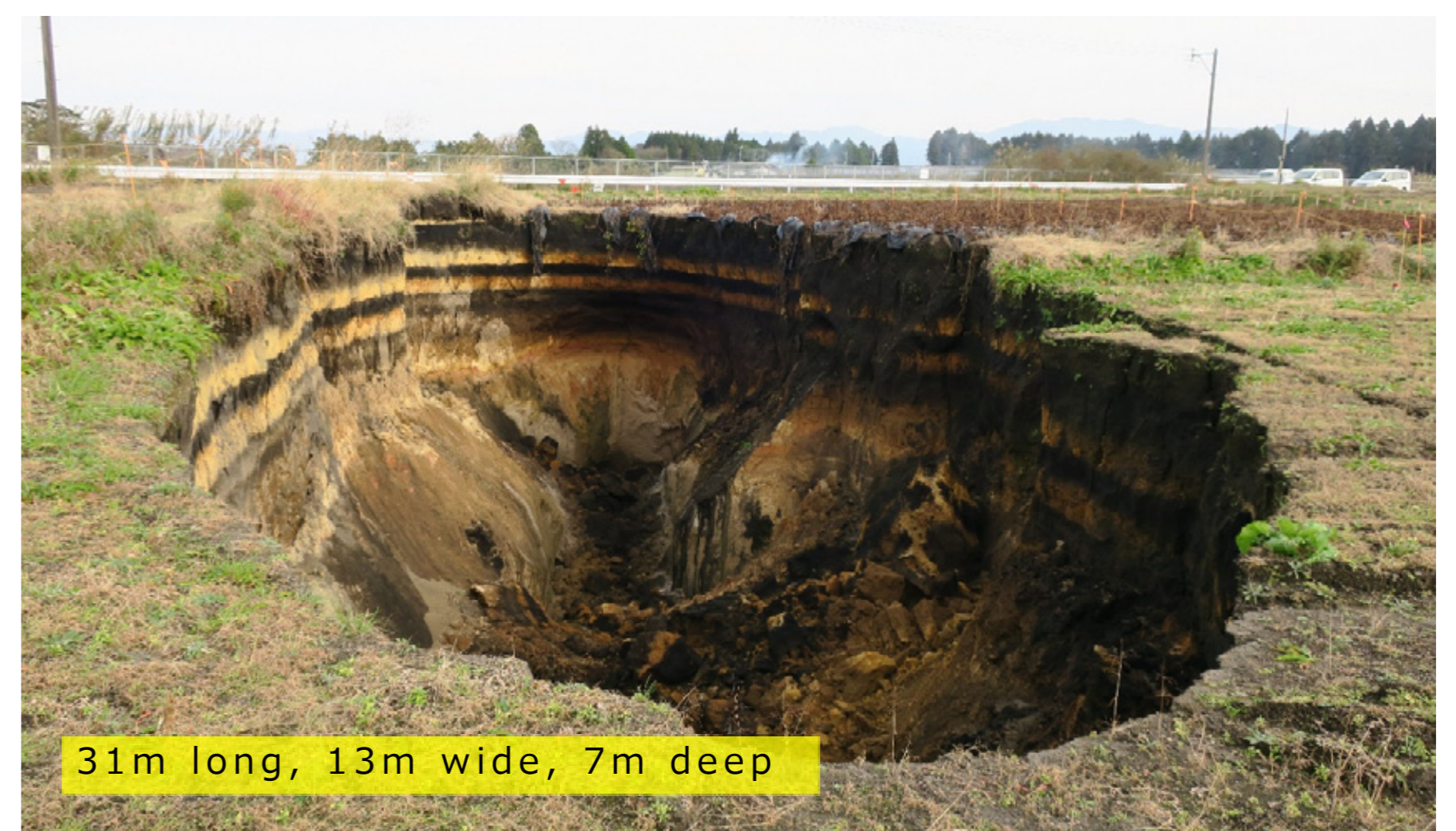
Sinkhole caused by internal erosion in volcanic "Shirasu" layer in Miyakonojo, Miyazaki (Sept. 2016)
