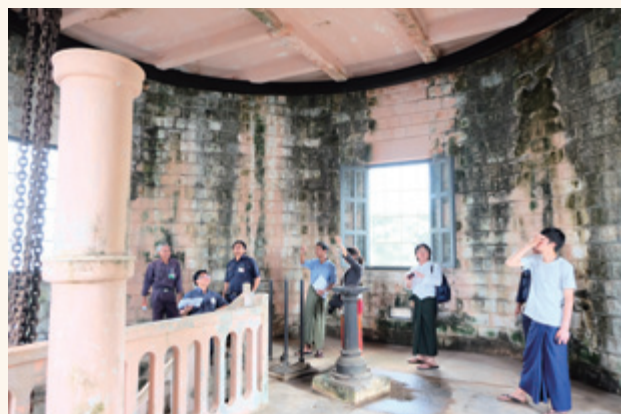
Visit to one of the old water facilities in the north of Yangon
