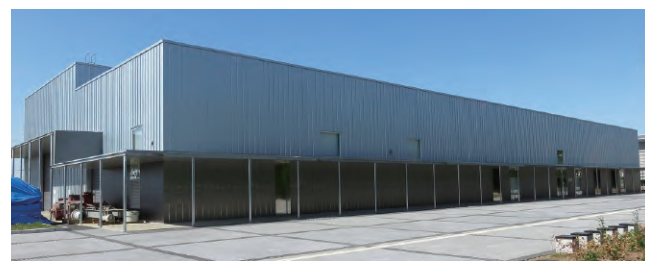
研究実験棟 II Research and Testing Complex II
