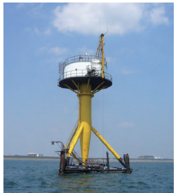
Microwave pulse doppler radar installed off Hiratsuka
