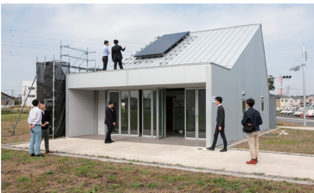
Test building constructed with developed renewable energy system
