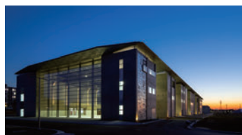
研究実験棟Ⅰ Research and Testing Complex I
