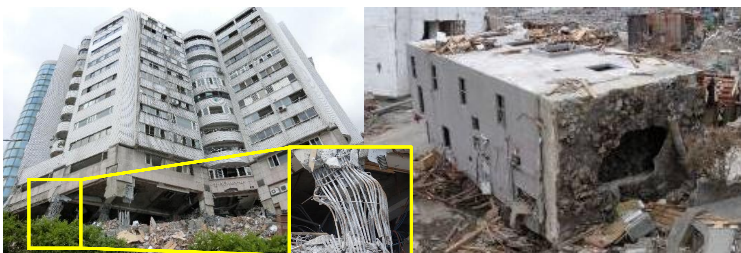
Building and its column collapsed due to earthquake
