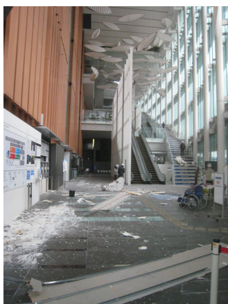
Great East Japan Earthquake
