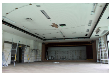
Ceiling reinforcement with cables
