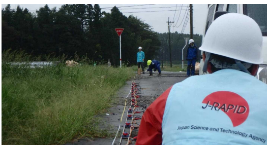
Field survey after geo-disaster
