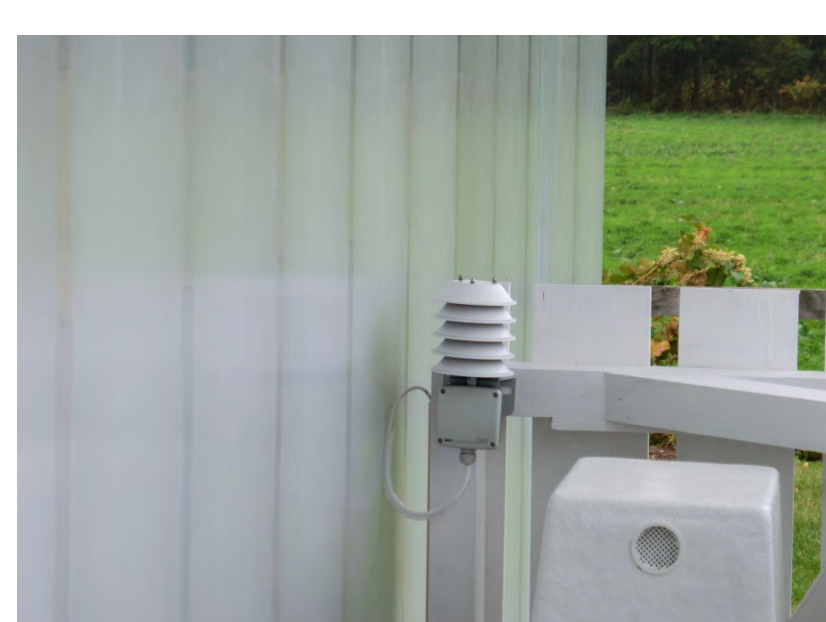
Outside air Thermal and Humidity sensors
