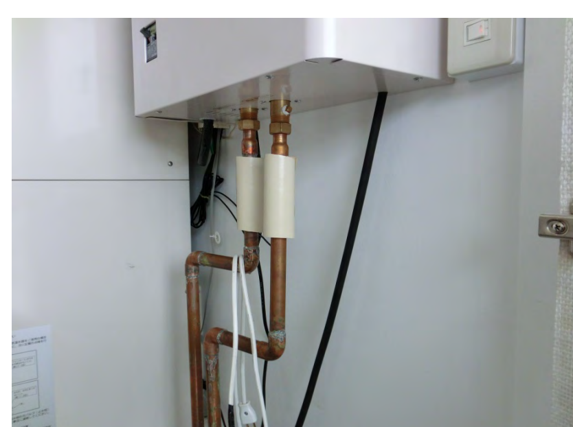
Boiler Thermal sensors
