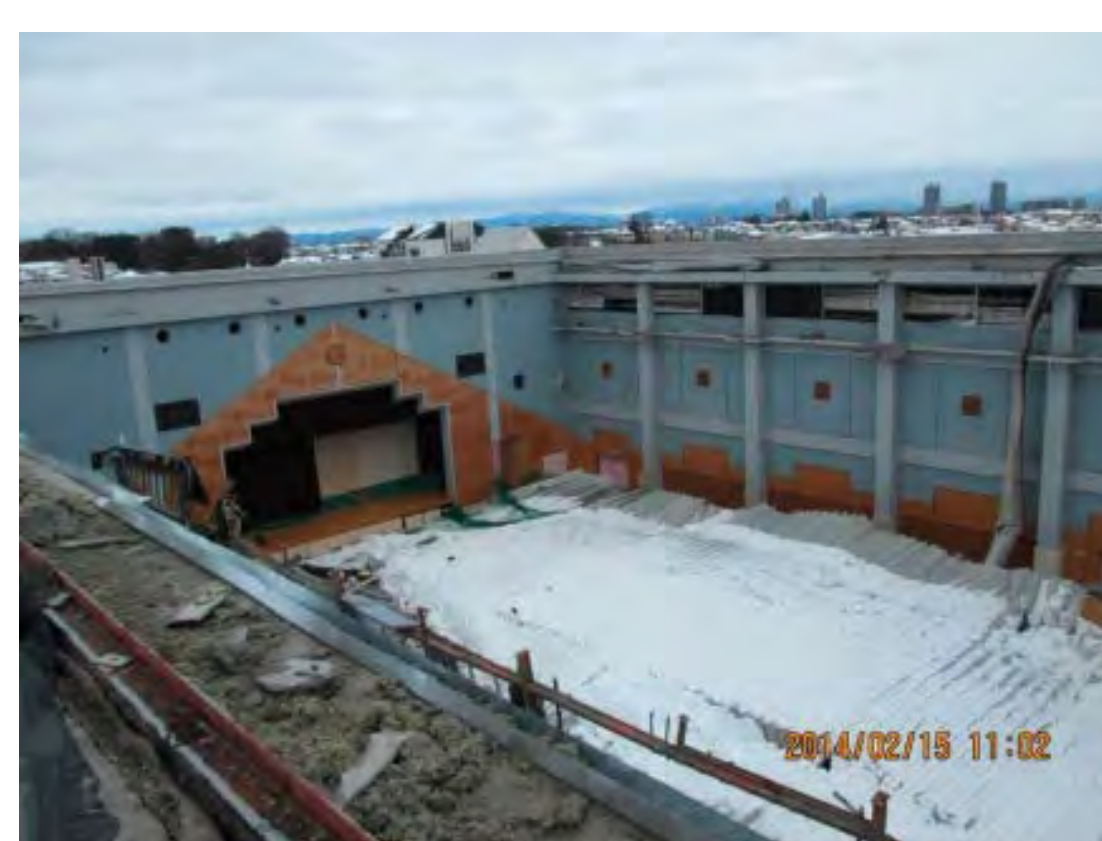
Roof collapse due to the heavy snowfall on Feb. 14, 2014
