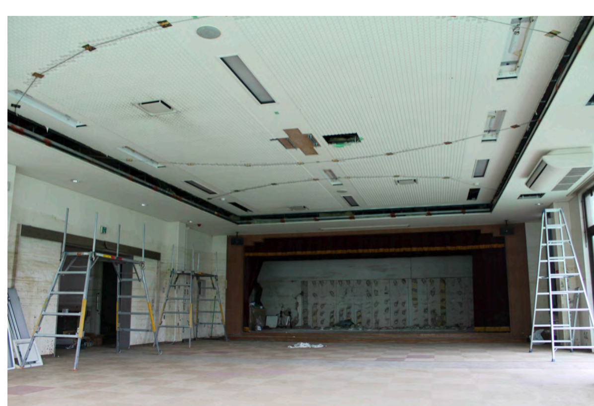
Ceiling reinforcement with cables
