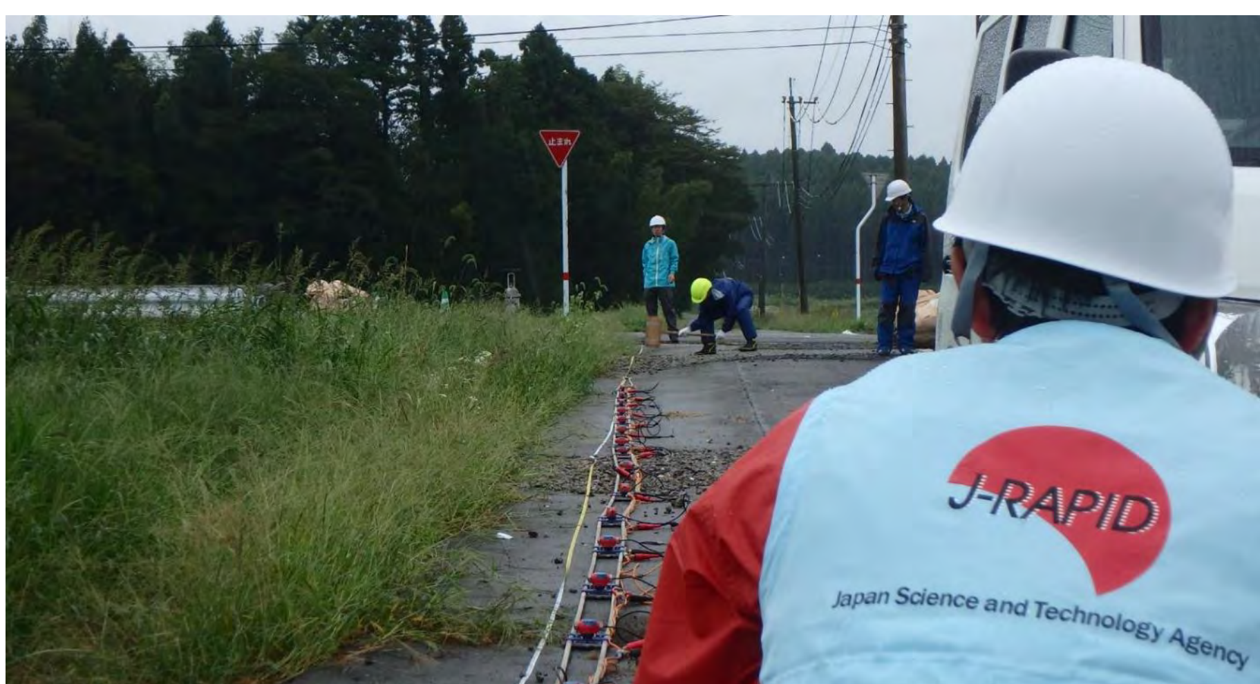
Field survey after geo-disaster
