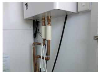
Boiler Thermal sensors
