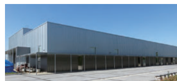
研究実験棟Ⅱ Research and Testing Complex II
