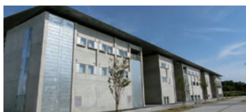
研究実験棟Ⅰ Research and Testing Complex I
