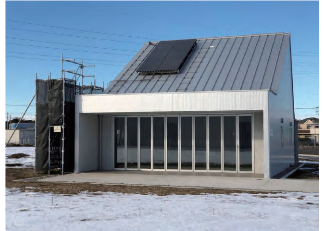
Test building with developed renewable energy system
