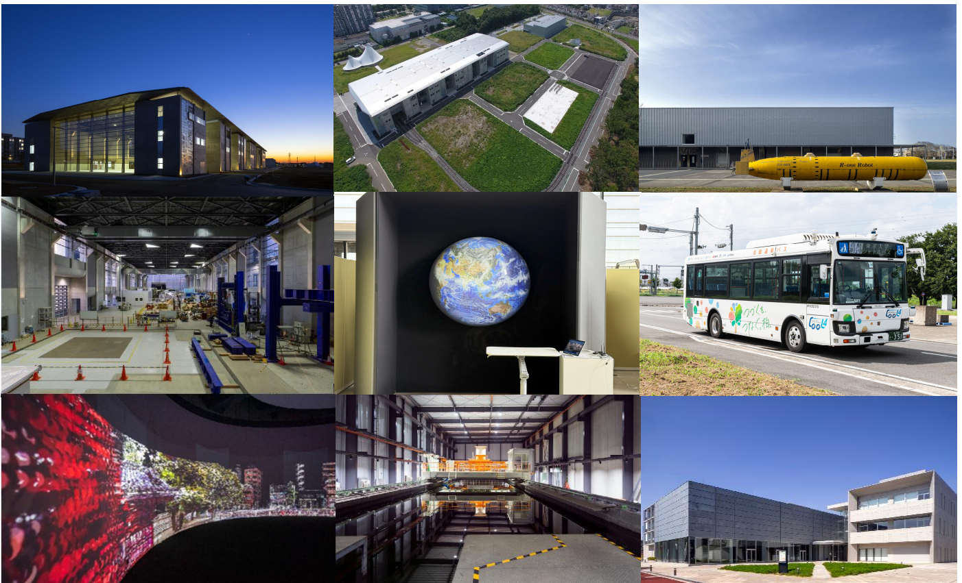
Research and Testing Complex I
