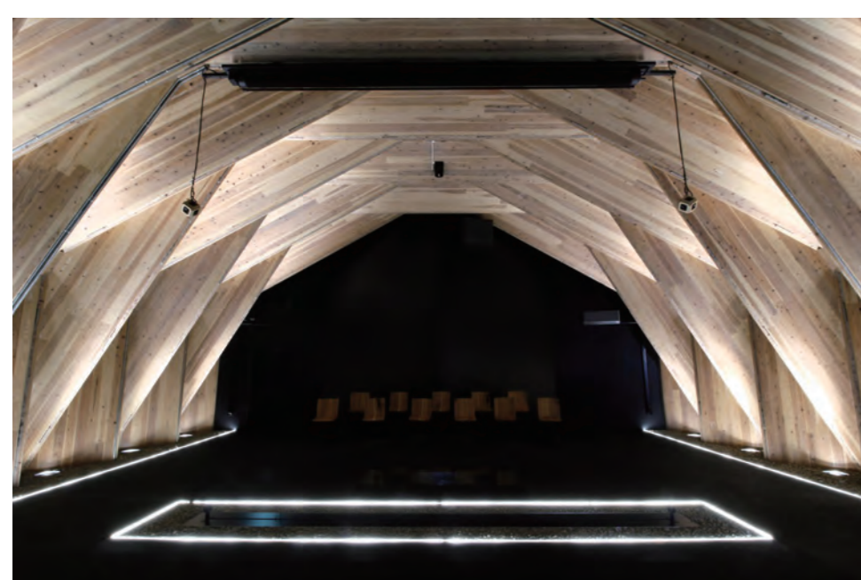
New Construction Method: CLT Folded Panel Construction
