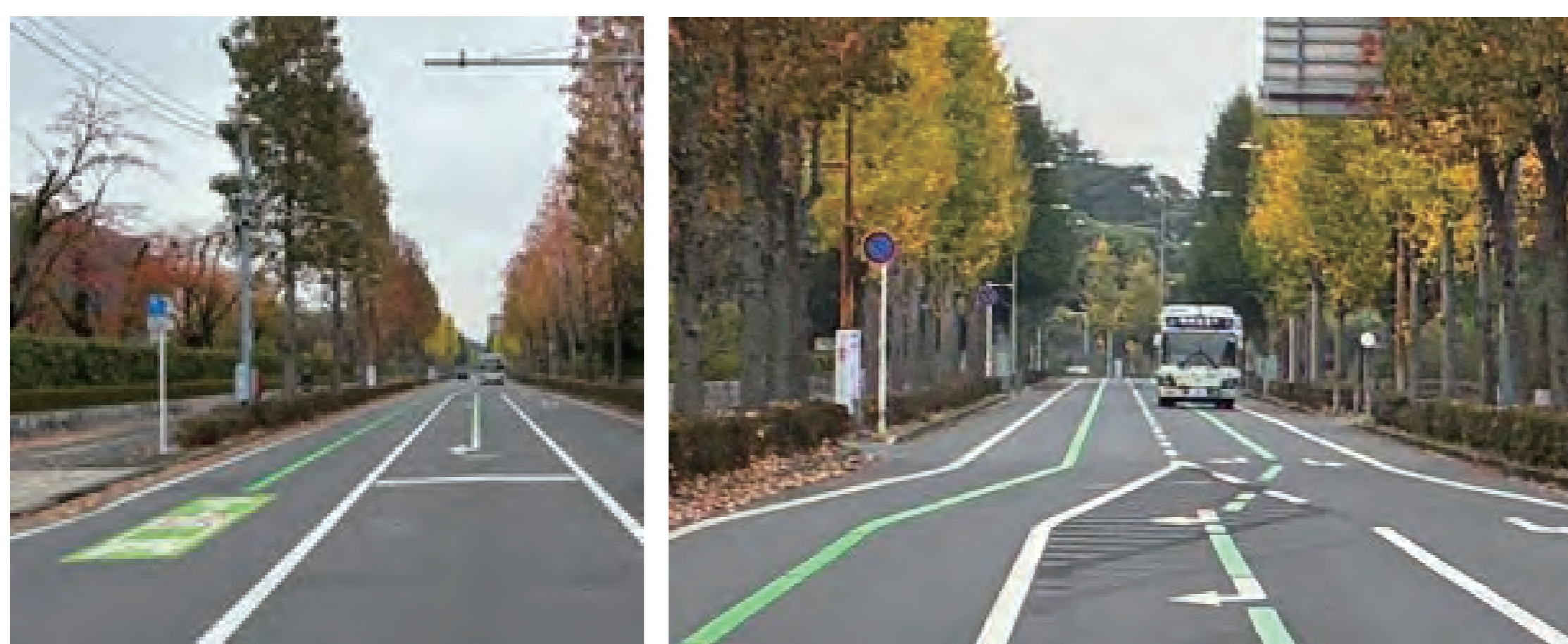
【Demonstration Experiment on Improved Stop Lines, Painted Medians, and Traffic Signs for Automated Buses】
