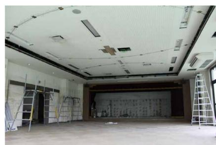
Ceiling reinforcement with cables
