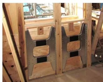
Seismic damper devices
