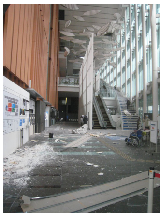
Great East Japan Earthquake
