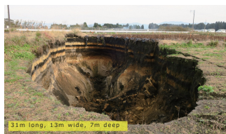
Sinkhole caused by internal erosion in volcanic "Shirasu" layer in Miyakonojo, Miyazaki (Sept. 2016)
