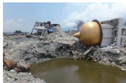
Field survey after geo-disaster
