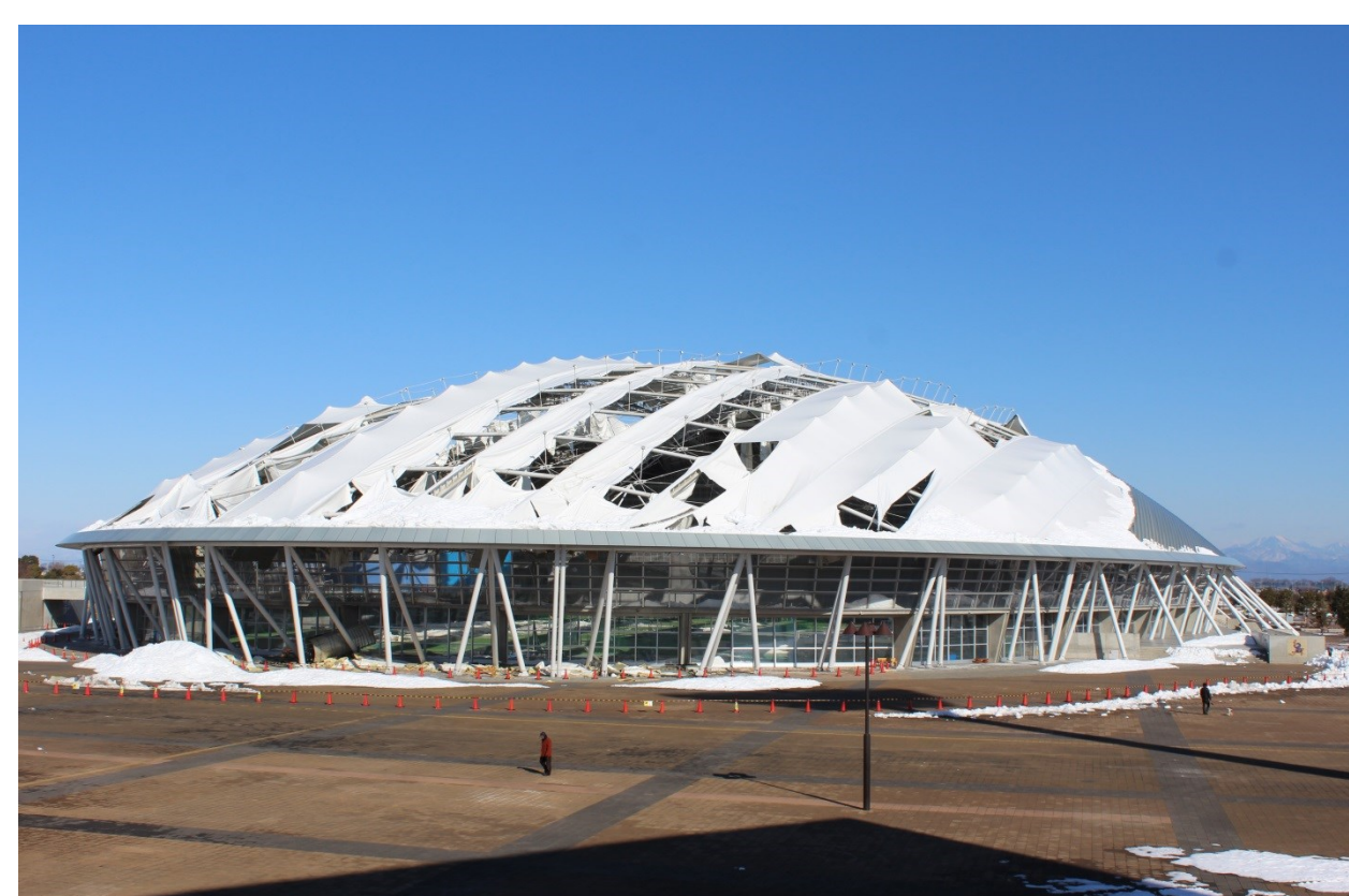
Roof collapse due to the heavy snowfall on Feb. 14, 2014
