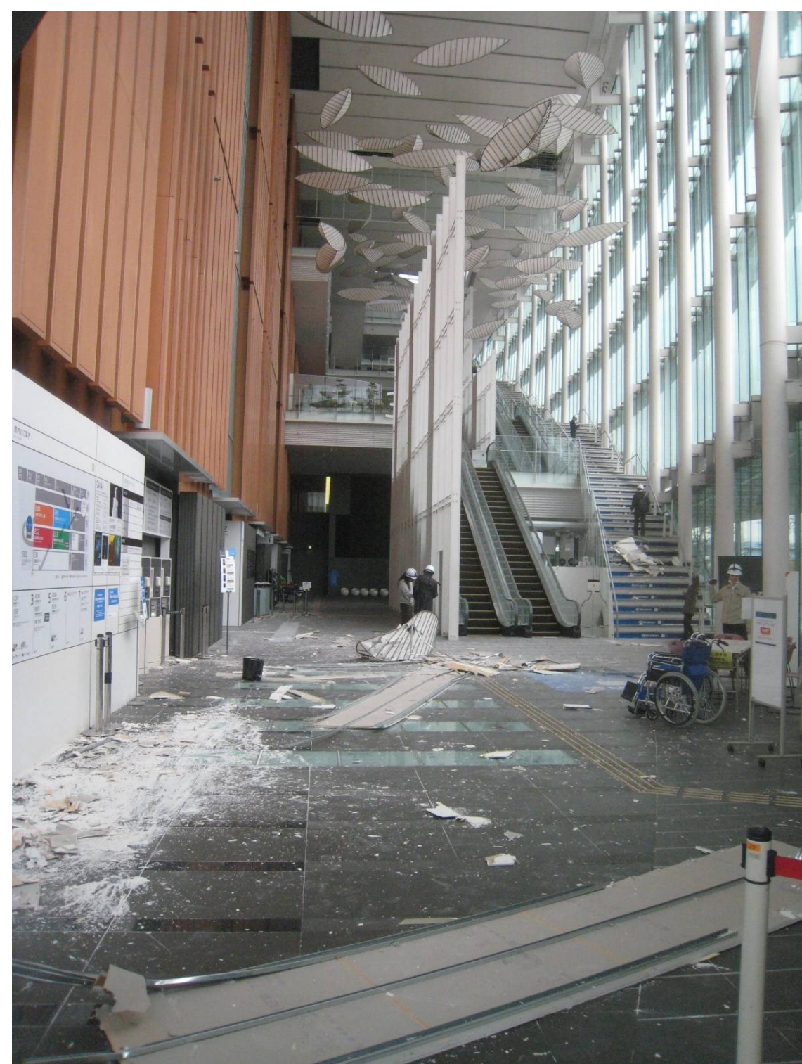
Great East Japan Earthquake
