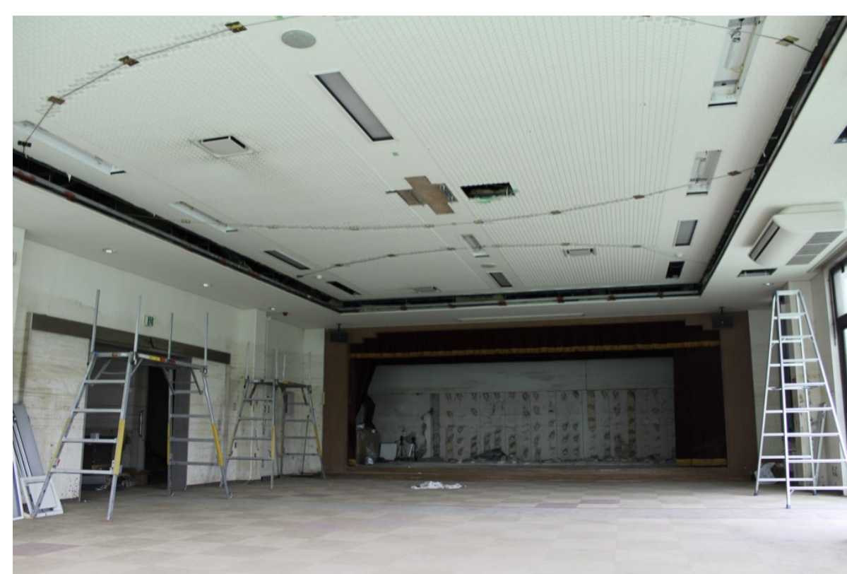
Ceiling reinforcement with cables
