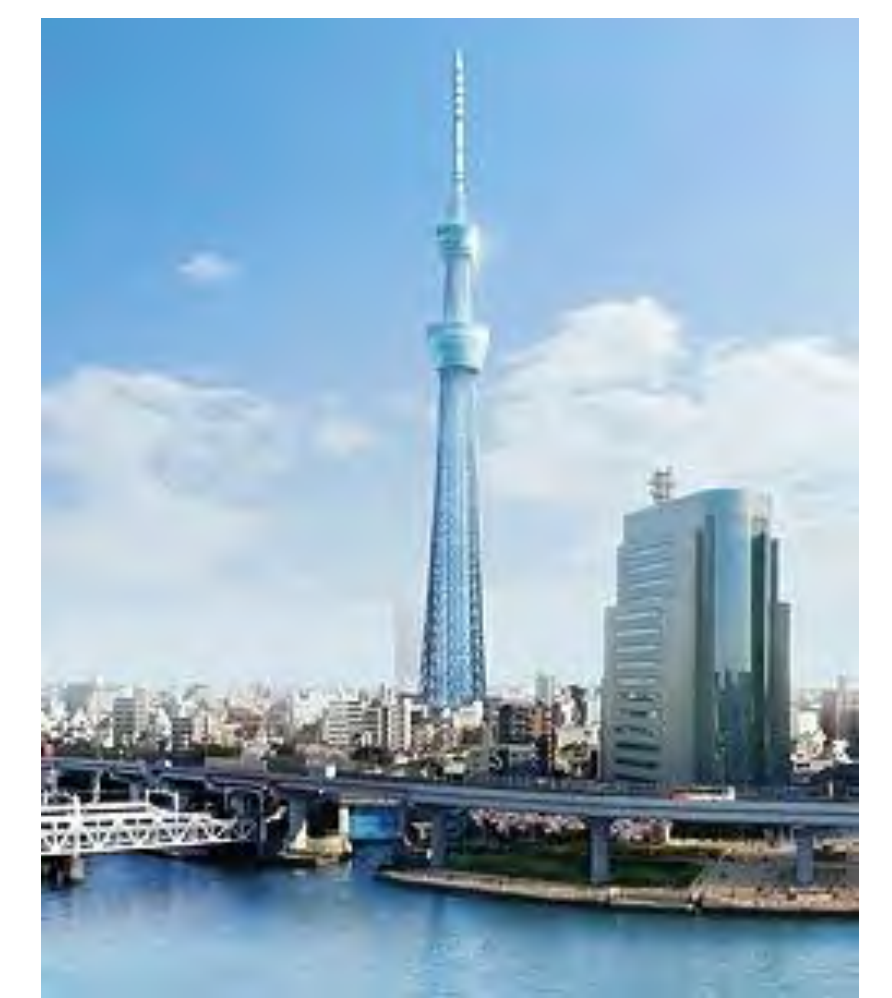
■ HVAC system using Pile heat exchanger
