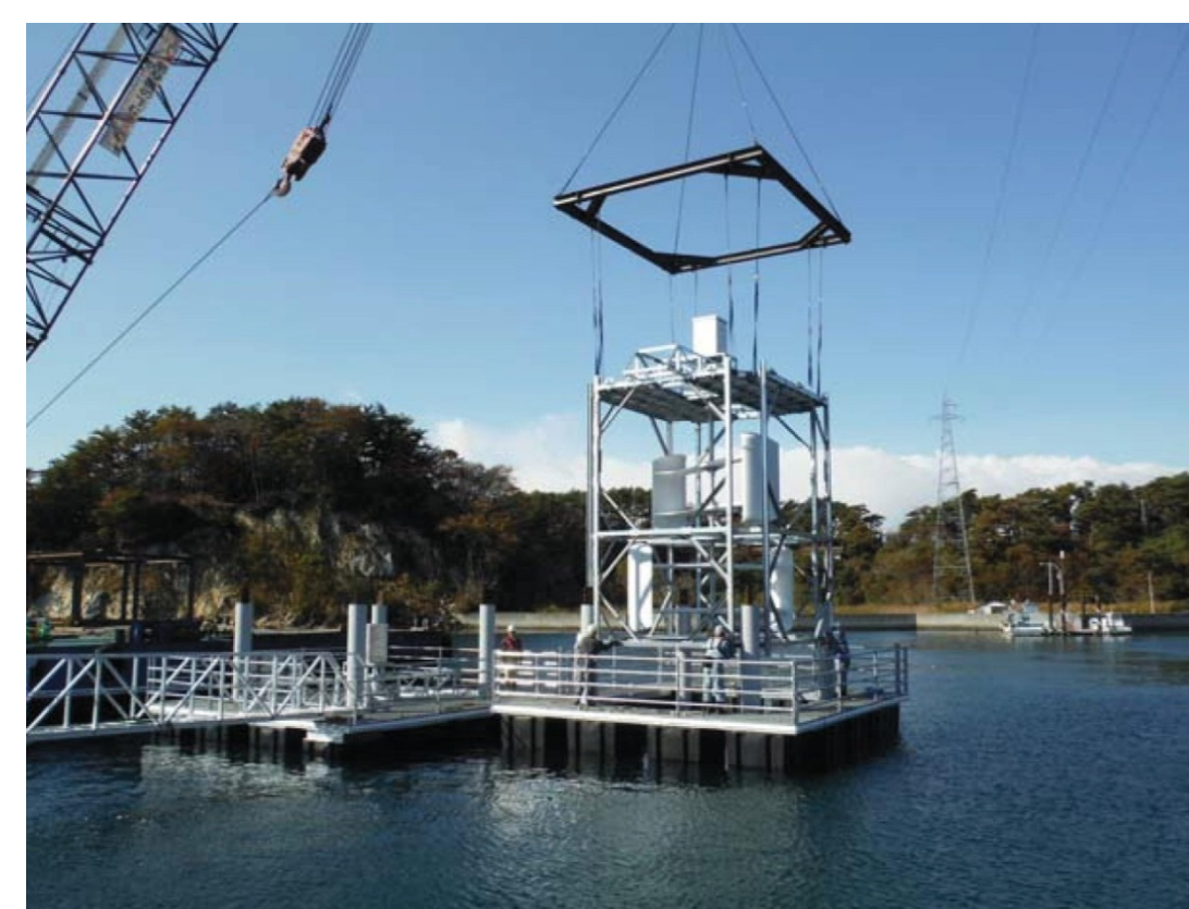
Installation of tidal energy converter
