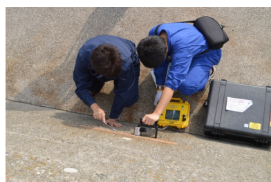
Fig. 3 Inspection of concrete coast levee
