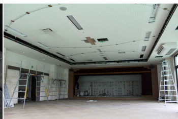
Ceiling reinforcement using cable
