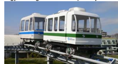
Mock-up of Rigid Frame Viaduct for Concrete Surface Quality Monitoring
