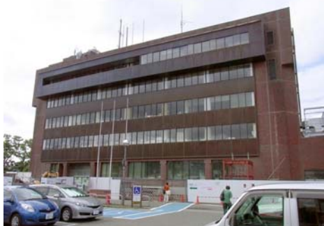
Susono city hall, Shizuoka
