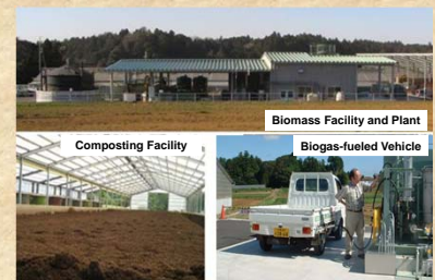
Biomass Facility and Plant in Katori City , Chiba Prefecture
