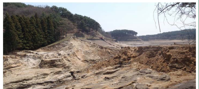
Dam-breaching at Fujinuma reservoir. The discharged water inundated downstream village (Sukagawa city)
