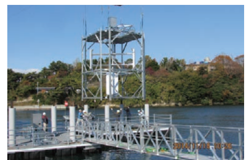
Tidal current power generator with two vertical axis rotors in Sabusawa channel in Shioyama city
