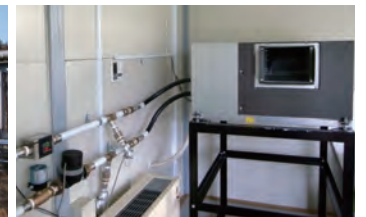
Cooling and heating heat pump
