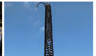
Geothermal heat exchanger
