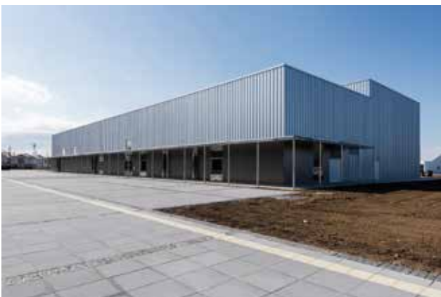
研究実験棟 II Research and Testing Complex II
