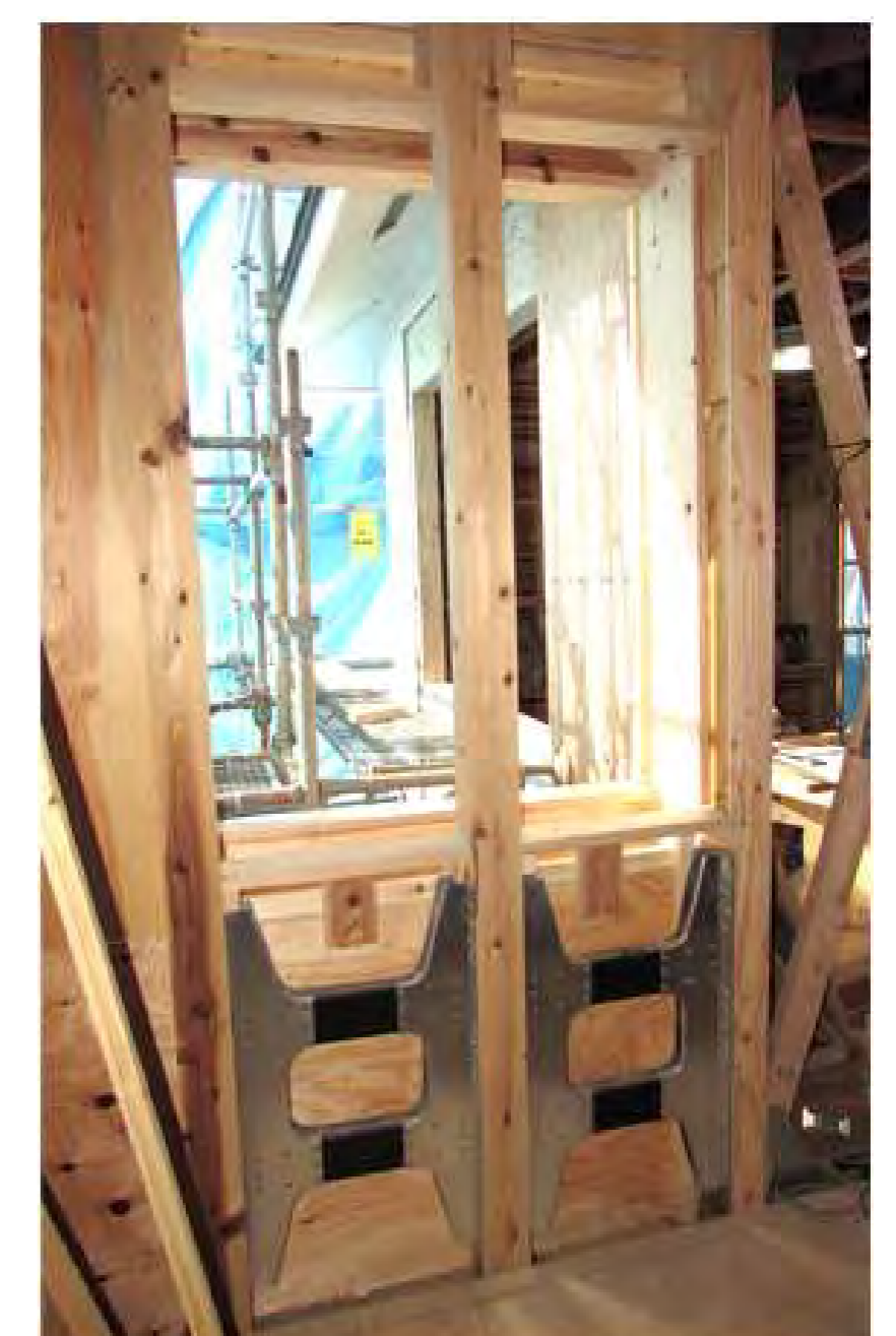
Seismic damper devices for narrow walls
