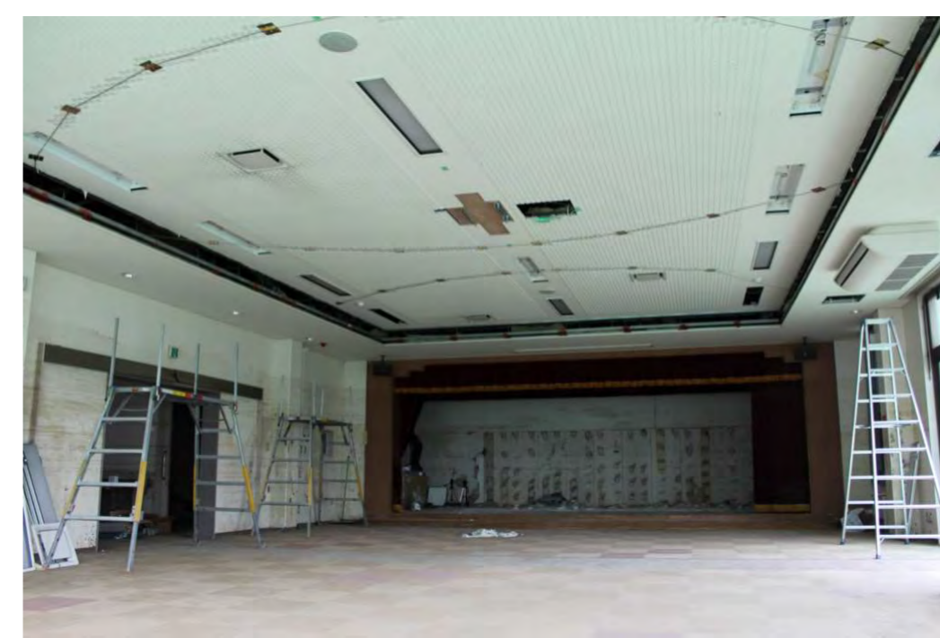
Ceiling reinforcement with cables
