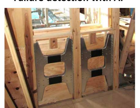
Seismic damper devices for narrow walls
