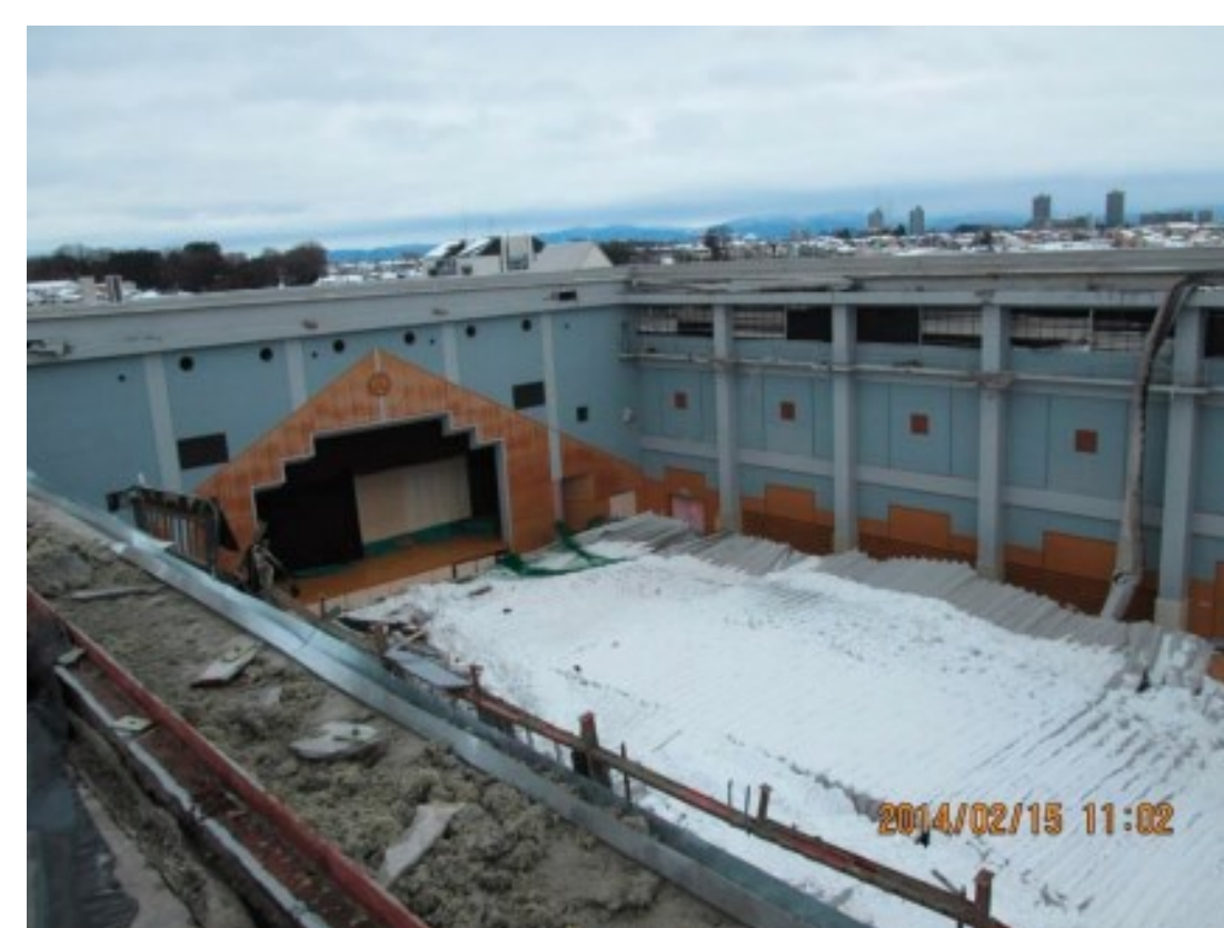
Roof collapse due to the heavy snowfall on Feb. 14, 2014
