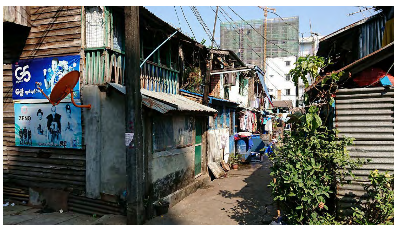
Existing wooden house in Yangon (Myanmar)
