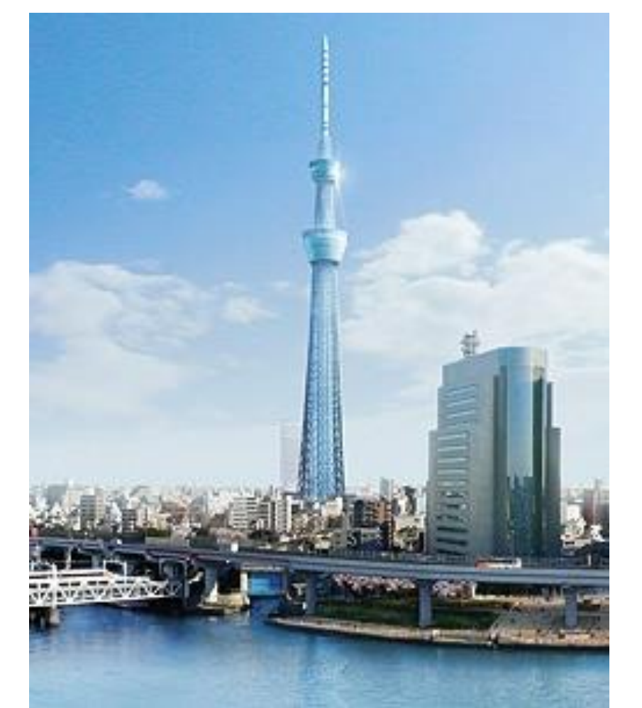
■ HVAC system using Pile heat exchanger
