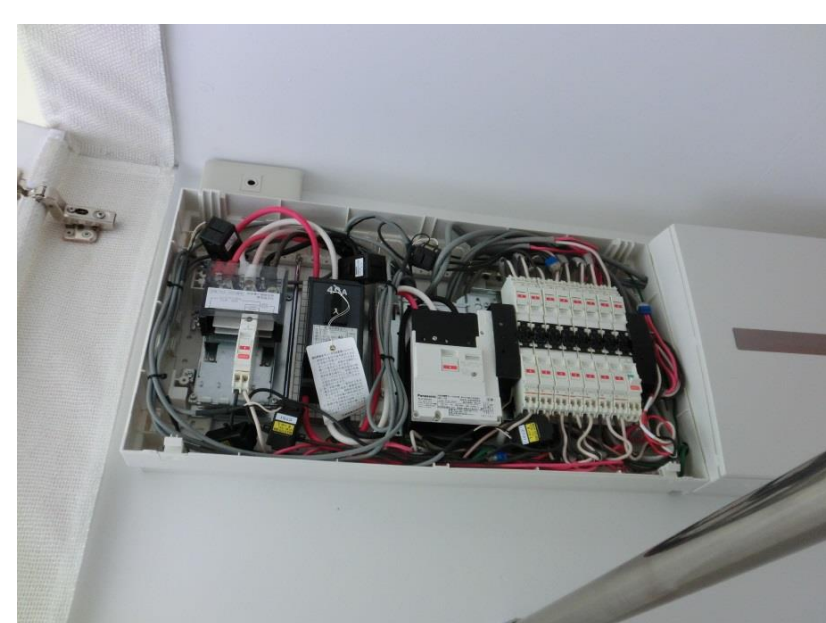
watt-hour meters 電力計
