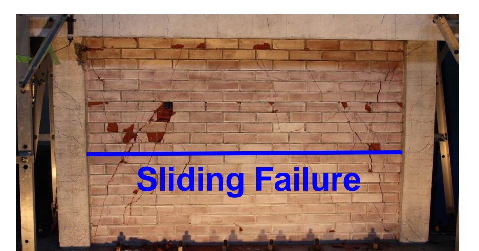
Weak Column Frame
