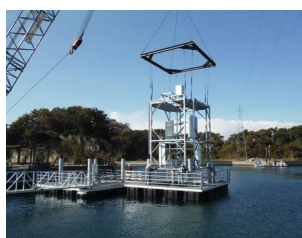
Installation of 5kW tidal energy converter
