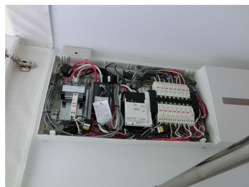
watt-hour meters 電力計
