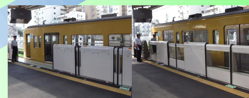
Variable-boarding-location-type Automatic Platform Gate
