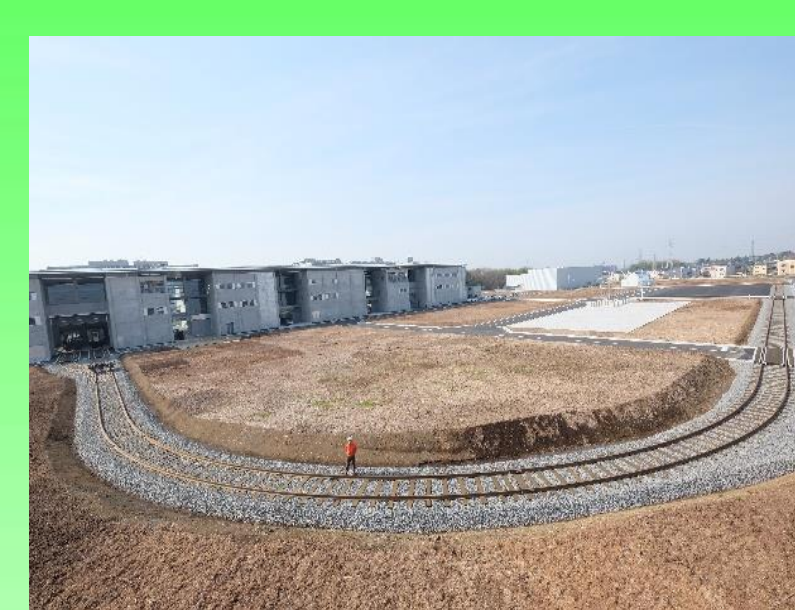
Full and Scaled Model Rail Vehicle Test Track for Innovative Designed Railway Truck
