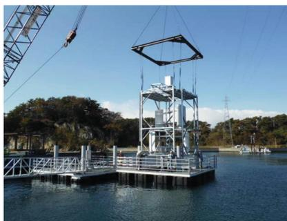
Installation of 5kW tidal energy converter
