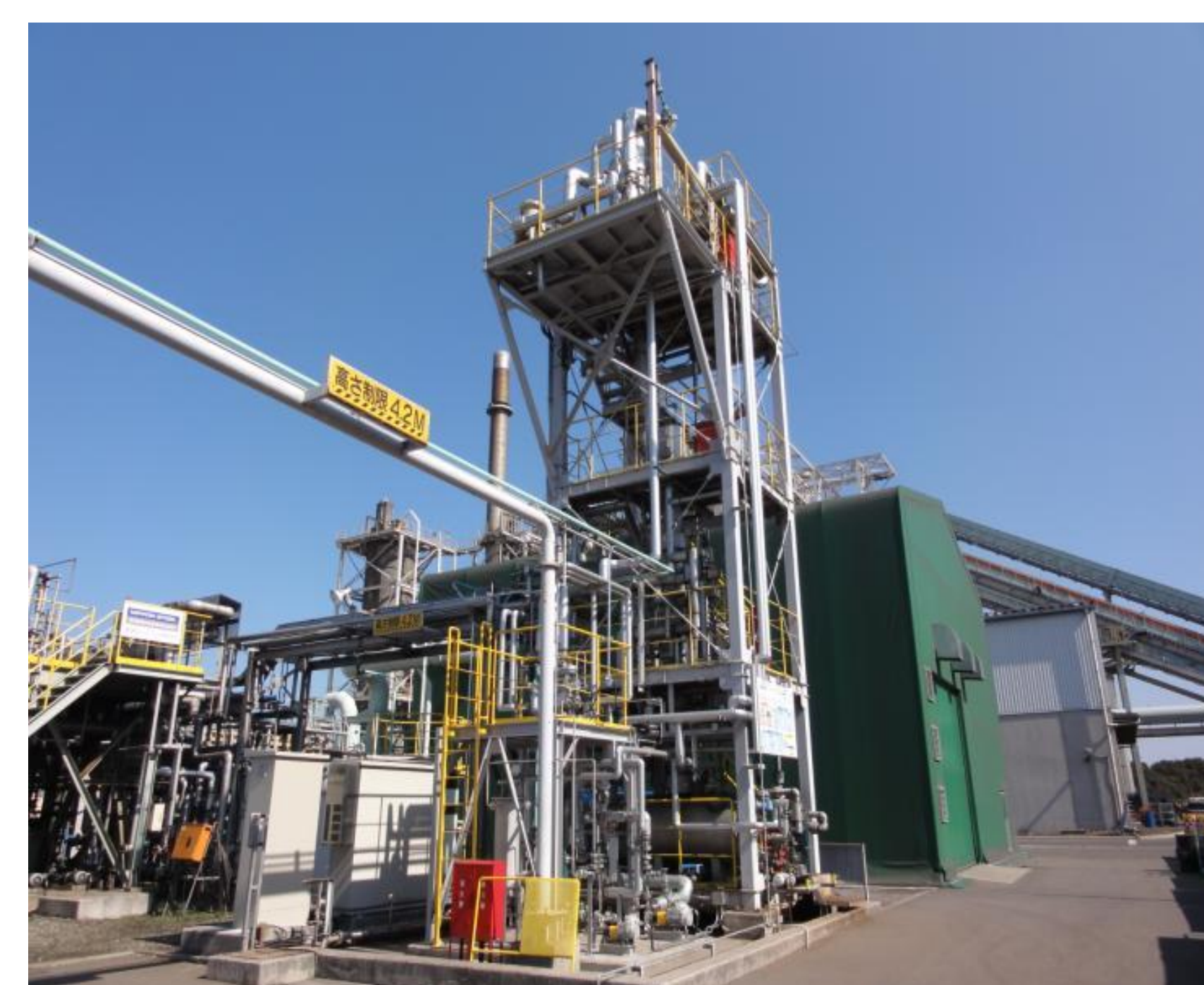
Pilot self-heat recuperative distillation for bioethanol Nippon Steel Engineering Kitakyushu Environmental Technology Center
