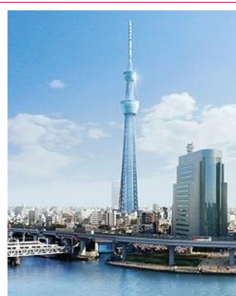
■ HVAC system using Pile heat exchanger
