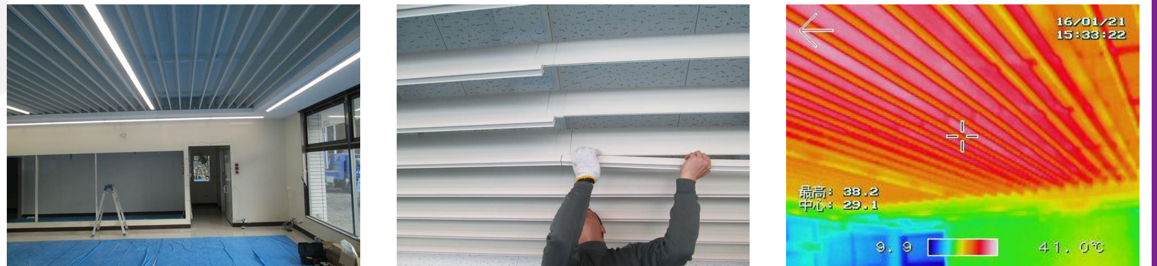
Pic.2 Environment and Energy Conservation store ▲ 70% energy saving (Target)
