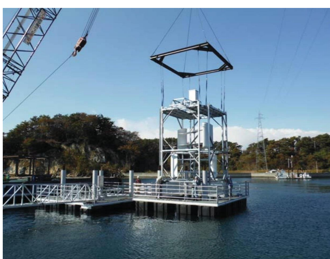
Installation of 5kW tidal energy converter
