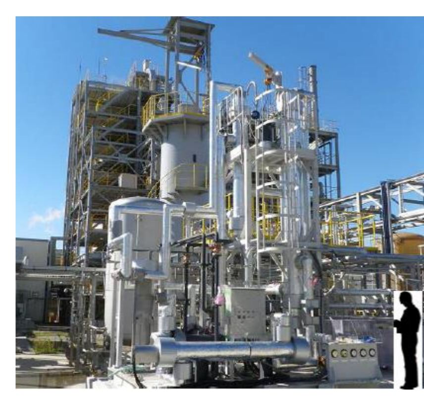
18Nm 3 /h-CH 4 demo. plant (Ref: Hitz)
