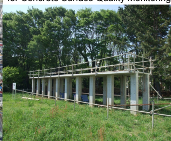
Mock-up of Rigid Frame Viaduct for Concrete Surface Quality Monitoring
